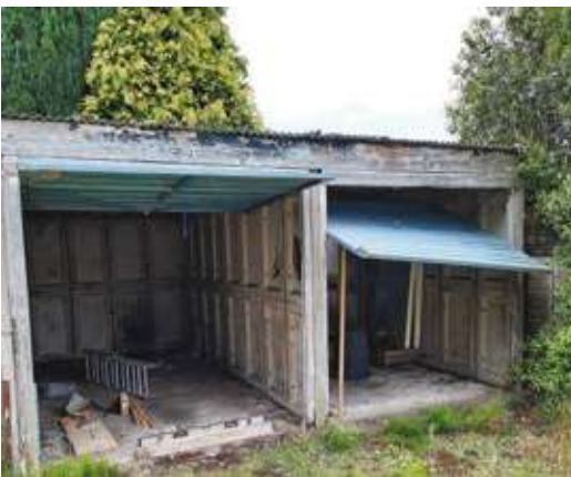
Hanson Garage Refurbs Pages 26-27
