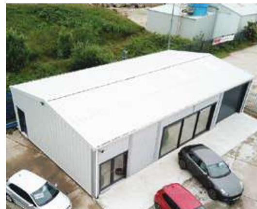
Hanson Industrial Buildings Pages 30-31
