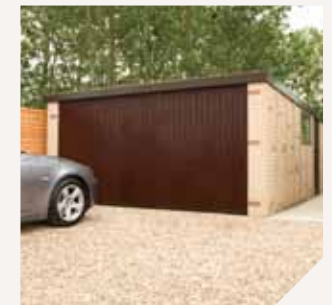
C Section galvanised rafters with Grafo-Therm treated galvanised roof sheet
