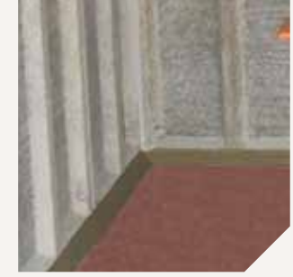
Sand and cement fillet
